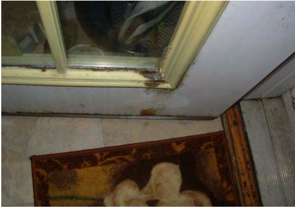
9. Spot door deterioration and rusting
