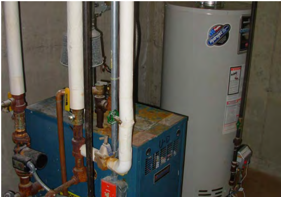
13. Heating and DHW equipment
