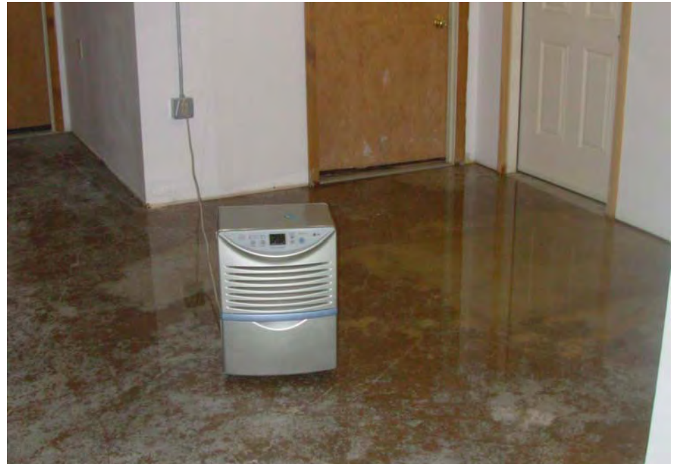
12. Areas of significant water infiltration in basements
