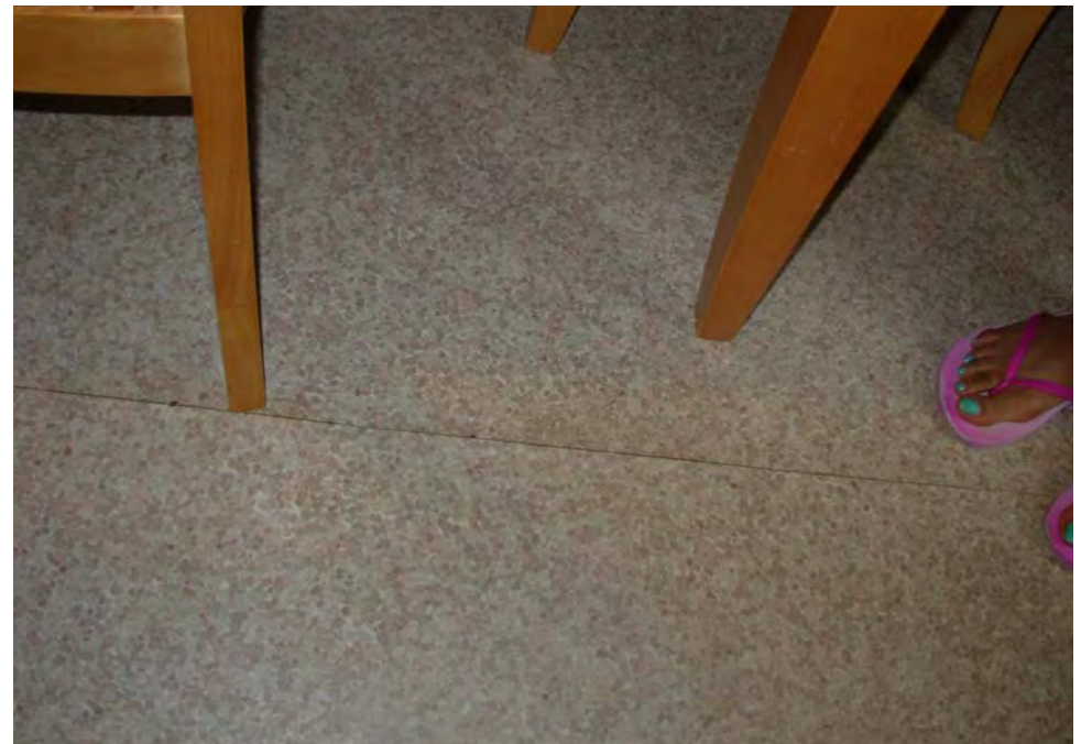
20. Unit kitchen and bath vinyl flooring with seam separation
